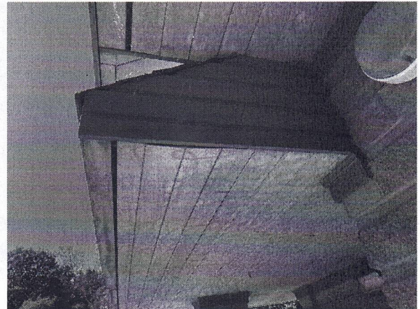
Photo 1.2: Exterior soffit – Discoloration, bulging, and open gap
