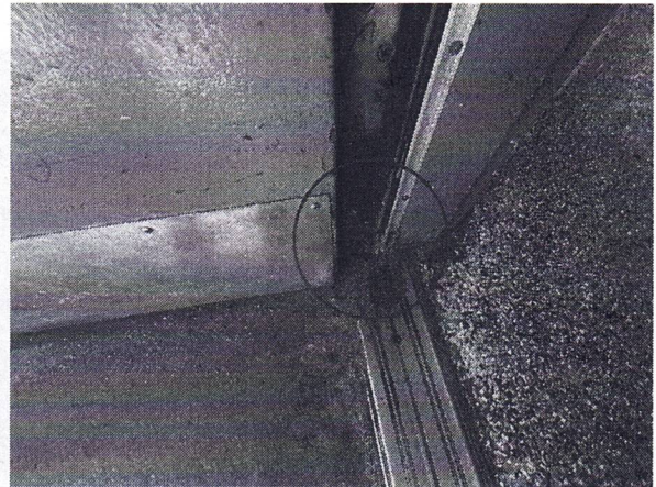
Photo 1.8: Washroom entrance door - Observed corroded frame
