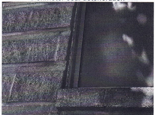
Photo 1.12: Perimeter seal deterioration
