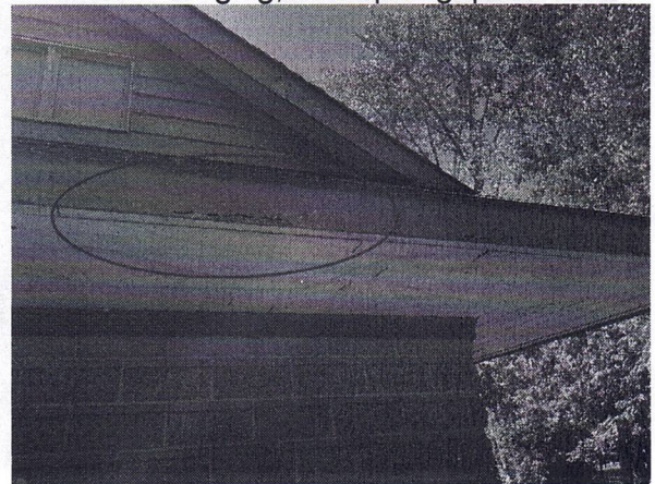
Photo 1.4: Fascia Board - Deterioration
