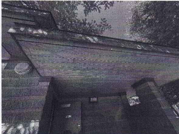
Photo 1.1: Exterior Soffit – Discoloration
